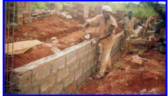
~ the walls go up
