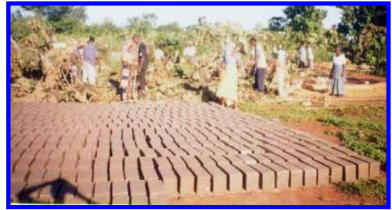
- assembling bricks for the school
